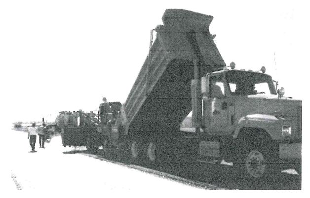
maintenance technique that consists of applying a layer of emulsified asphalt and then aggregate to a road's surface. This treatment acts to preserve the pavement by protecting the surface from degradation caused by sun and moisture and extends the pavement life through the addition of a wearing course.
